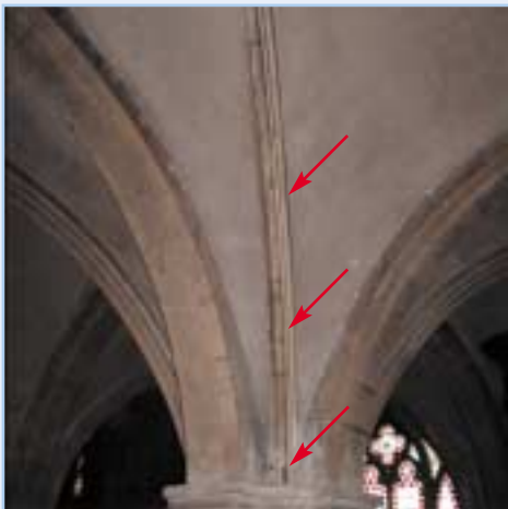
Optical Strand in a church vault.
