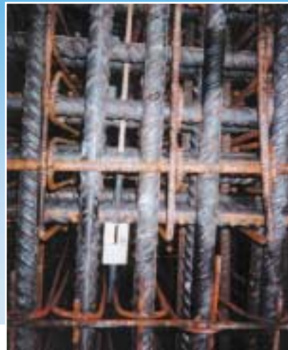
Optical Strand in a reinforcing cage.
