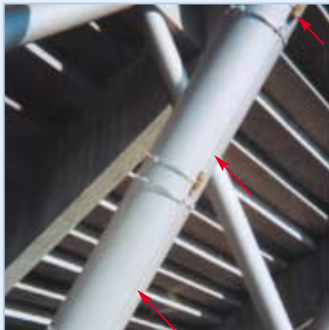
Optical Strand on a steel prop.
