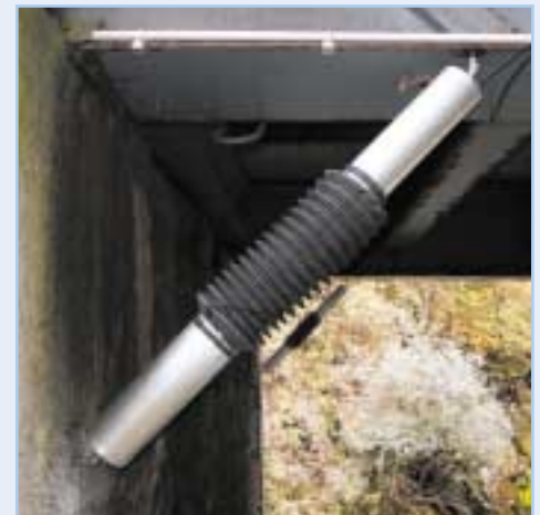
Detailed view of an EX-Large, zero-play attachment.
