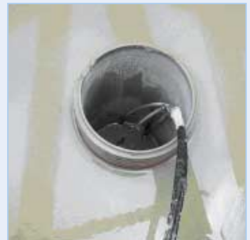
Optical Strand in injected bores.
